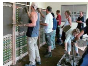
Building an earthen wall
